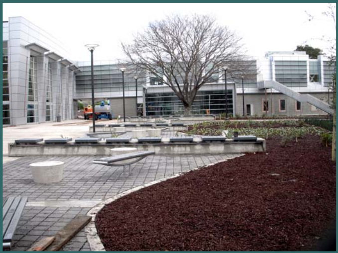
Back of New CSSC Building.
