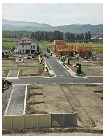
Construction Adjacent to LPC Campus
