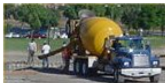
Construction Work at Chabot Campus
