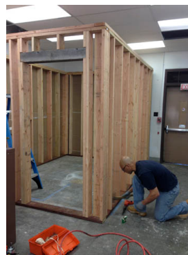
Storage Room Construction
