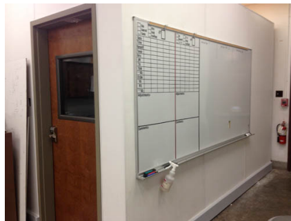
Completed Temp-Controlled Wine Storage Room
